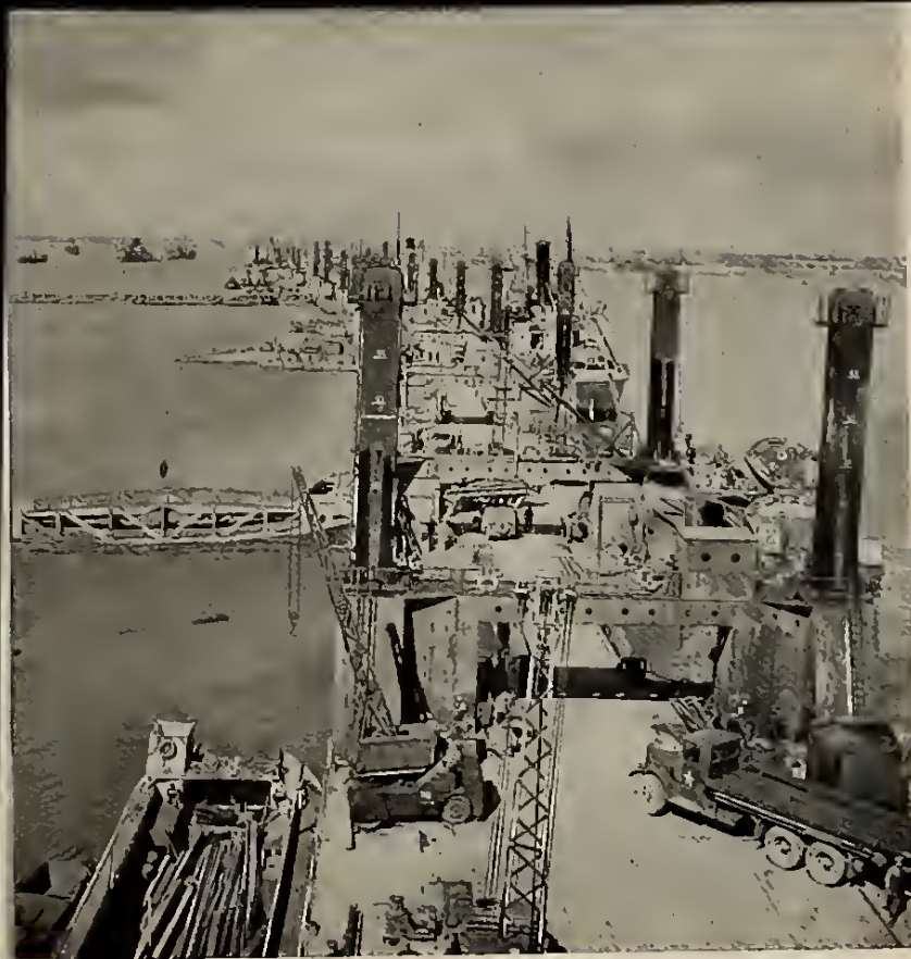
7. Here is seen a row of seven pierheads, joined together by bridges to form the wharf. Note the markings on the legs indicating the depth of the water.
